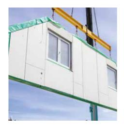
Modular housing can be tested during its development stage for structural and environmental performance – there are a myriad of different test techniques that will prove the modules or panels are fit for purpose when constructed in the factory. The unknown is the effects of transporting the panels or modules to site.
